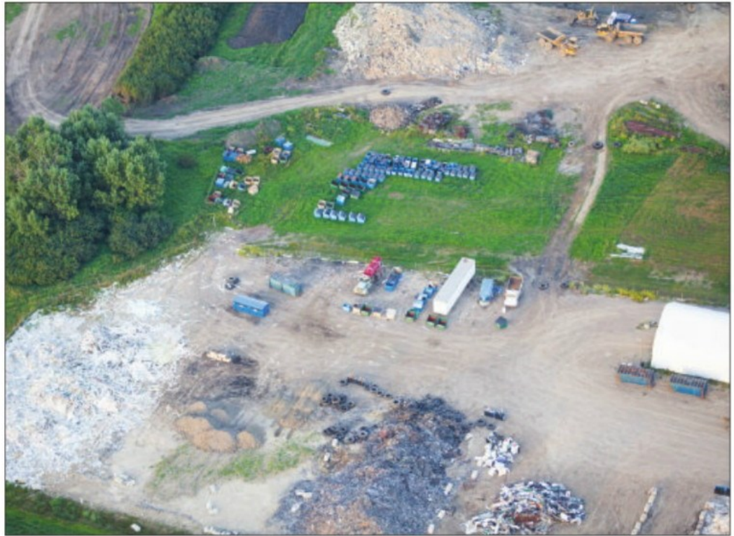
Mountain View Waste Commission landfill just north of Didsbury.
